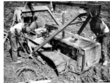
Muskegs are like a muddy version of quicksand. A vehicle would pass through a muskeg once, but within a short time, the area would turn into liquid mud, losing strength. Once caught, a vehicle had to be pulled out. (Photo and caption courtesy of Missouri University of Science and Technology 2014.)
