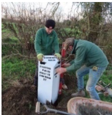
Replacing a Alderminster milepost Photos: Mike Buxton
