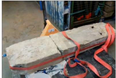
Resin bond repair to join the Milestone back together (14 October 2019)
