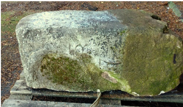
Damaged Ferrybridge face
