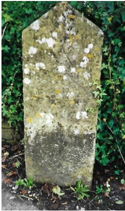
Milestone before restoration
