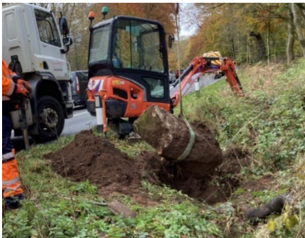
CU_CLCN12 being removed Photo: Terry Moore
