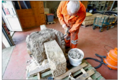
Removal of the concrete collar using a cold chisel (12 July 2019)
