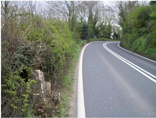
Figure 8: SX398611 A388 S of Hatt damaged in 2008, later destroyed in 2014.
