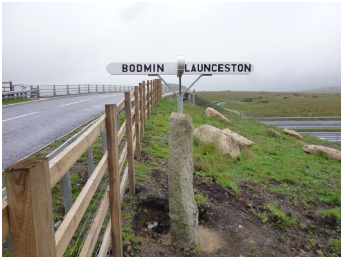
Figure 15: SX136736 A30 Temple Moor. Restored fingerpost with new ironwork and arms in August 2018.
