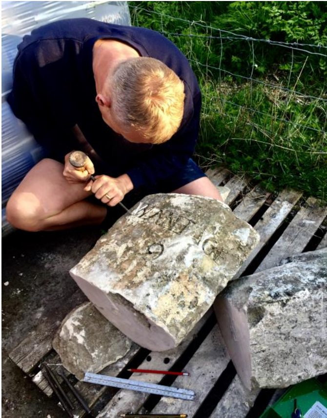
Figure 4: Blewbury milestone in process of repair by stonemason Ryan Morris. Photo: Emily Tucker.
