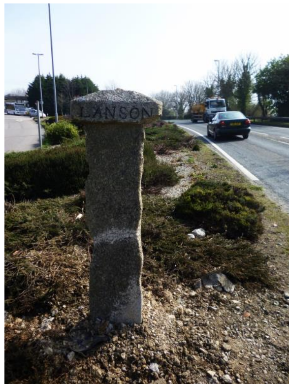
Figure 6: The guide stone repaired and re-erected the wrong way round in February 2015.
