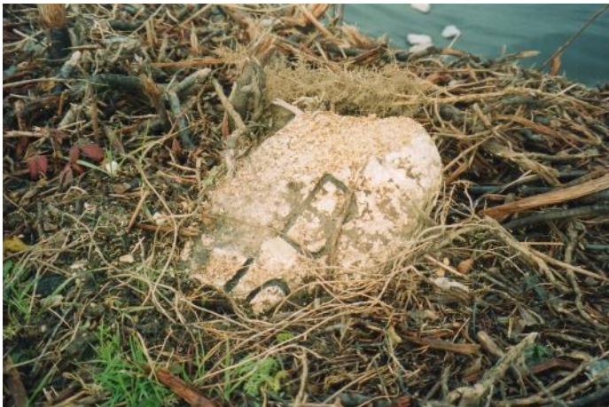
Figure 3: January 2006. Milestone spotted in debris of hedge removed during road improvements. SW939602, A30 Grade II listed St Columb, List Entry Number 1327412.
