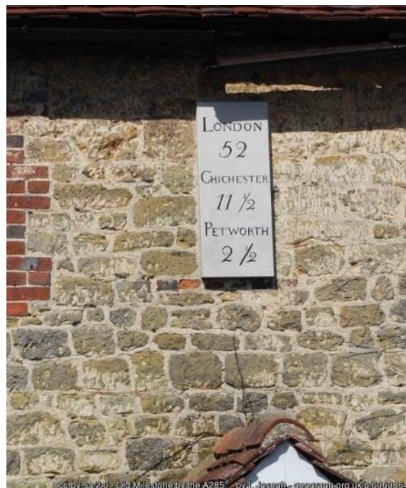
Figure 3: Restored mileplate near Petworth, SY 96356 18046, SX LMP 52.
