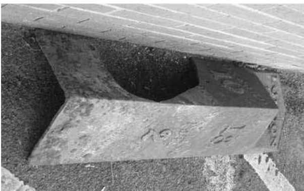
The Shillingford milepost [Oxon Highways photo]
