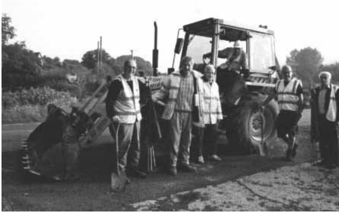
7.30 am on a Sunday morning. Members of the Worcestershire Group meet with local parish councillor Bert Bradley and prepare to raise the sunken Ham Bridge milestone in preparation for the attachment of a new plate made by local member, Martin Horwood. Photo by Peter Willis
