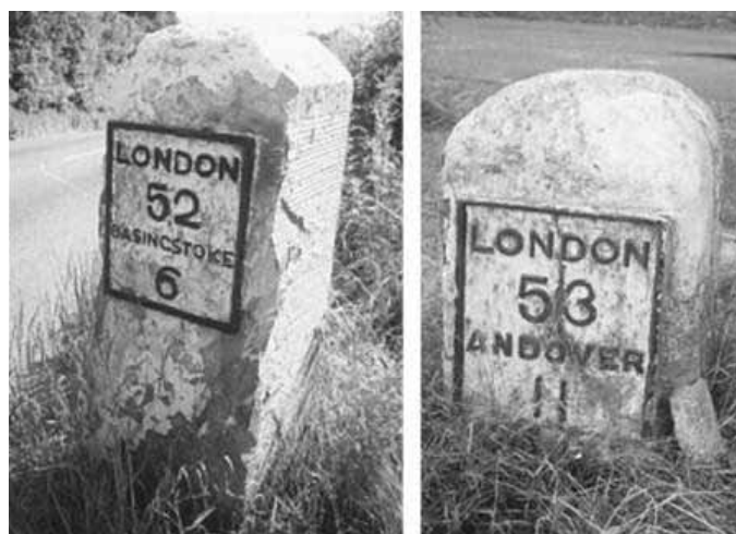
The 'LONDON 52 at Deane (BAAN06) 'LONDON 53 at Overton (BAAN07) before the loss of their plates. [Photos Keith Lawrence]
