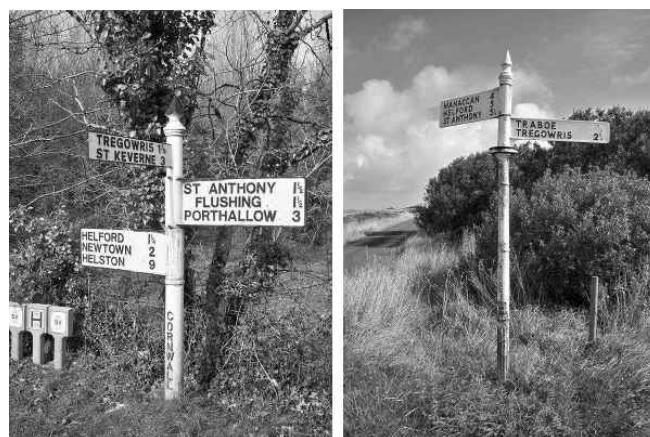
On The Lizard. [Left] Alloy fingerpost on the Lizard (test with a magnet). Top arm is a plastic replacement. [Right] The pillar and finial are late C19 made by Toy of Helston although the arms are 1930s replacements made by IRS Ltd.
