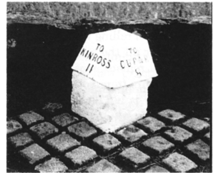
One of a number of designs of Fife milestones. The cast iron cap on this one is attached to a whinstone pillar. Note the latest experiment in weed control
