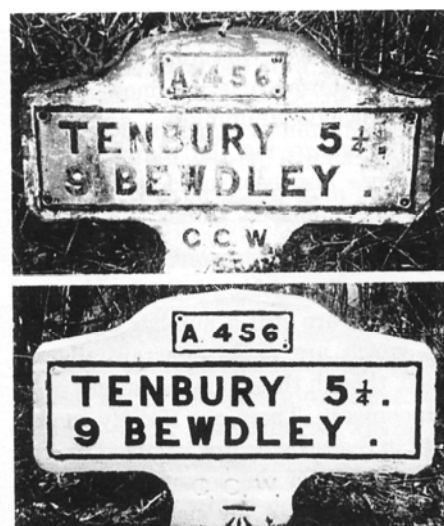
From Worcestershire comes an example of renovation of one of the concrete Bradley stones with two cast iron plates.
